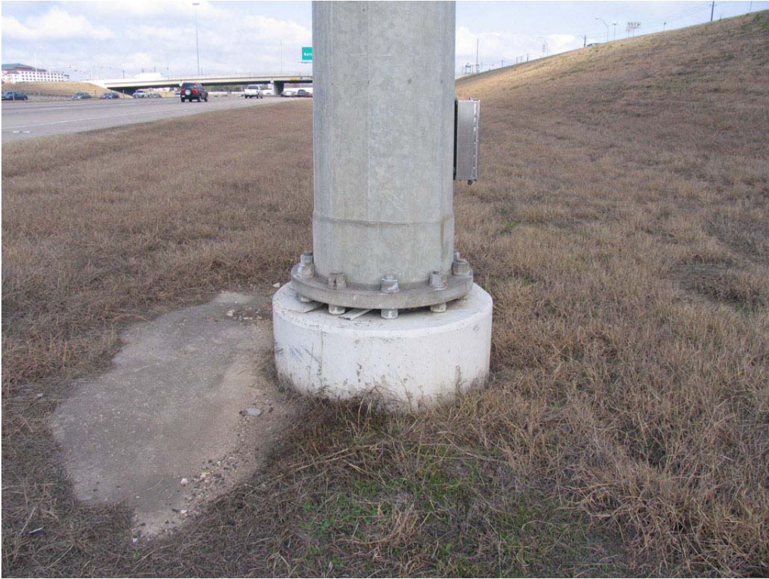
Figure 1.3: High-mast lighting tower foundation
