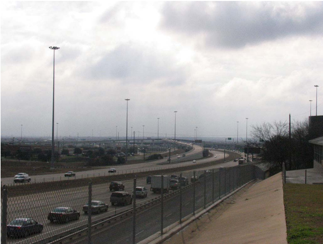
Figure 1.1 High-mast lighting towers at a highway intersection
