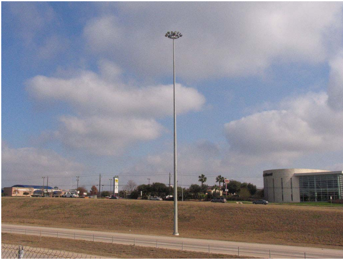
Figure 1.2: Typical high-mast lighting tower
