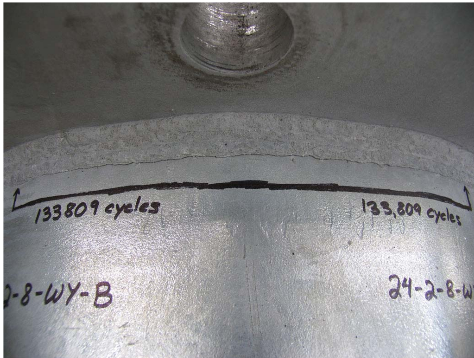
Figure 5.3: Typical failure of Wyoming full penetration weld connection
